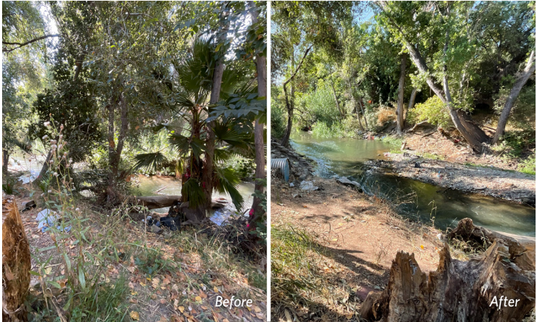
Vegetation was removed from the east bank of Guadalupe River downstream of Coleman Avenue in San José to restore the stream's design flow conveyance capacity.
